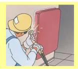
1. Position the door. Place the door frame at the appropriate site and tack weld it into position. Then solidly weld the frame to the surface.
