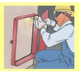
2. Cut the inside hole. Open the door and carefully torchburn the center to create the access area.
